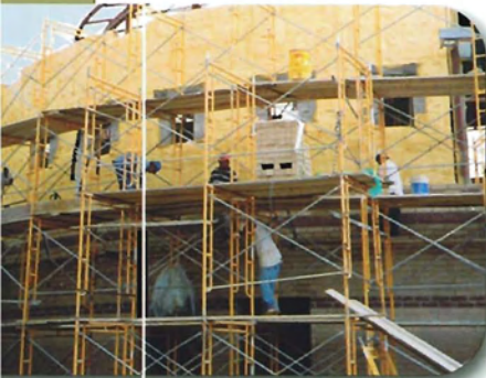
< InsulBloc adheres to CMU, poured concrete, primed steel, wood and most other construction materials.
