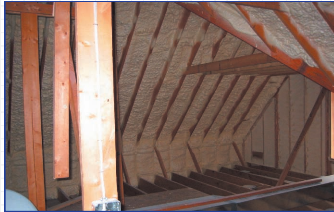
Icynene® adheres to common construction materials and maintains its efficiency with no loss of R-value over time. Icynene® does not shrink, sag or settle.
