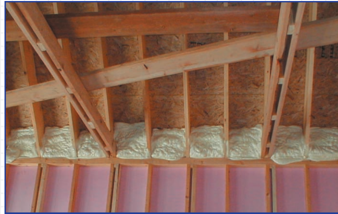
R-18 is sprayed into the rim joists of the basement area to prevent warm, moist air from coming into contact with cooler wall services, minimizing the potential for condensation.
