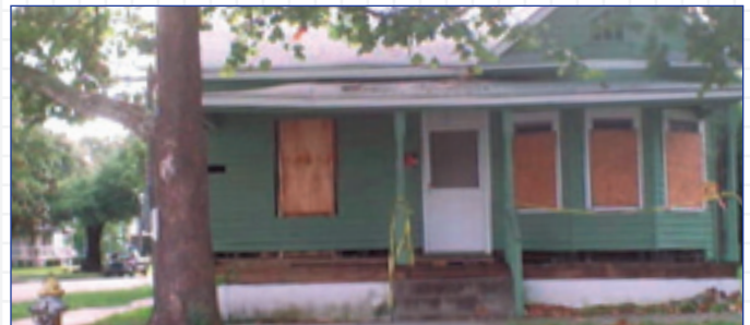
Icynene®, a high-performance insulation, was selected to address the homeowner's strong allergic sensitivity and reaction to mold and mildew.
