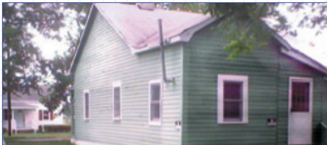
This abandoned home in Wilmington's historic district was gutted and restored to meet Energy Star™ standards.
